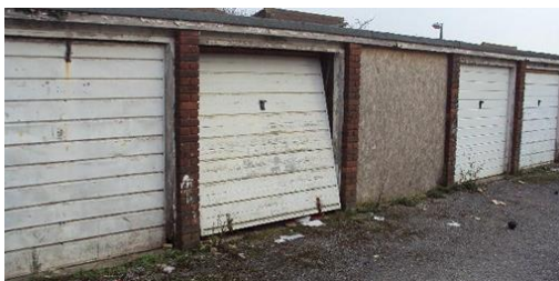
Before: Flint Close garages
